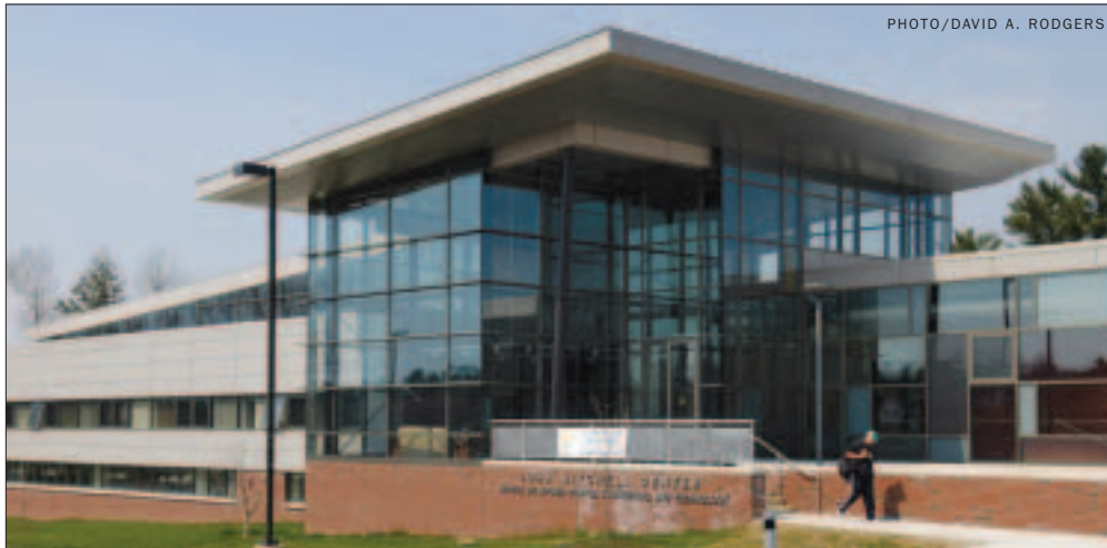
Push and pull: Kevin Whitney says getting LEED certification for this USM building meant going back and forth with the U.S. Green Building Council
